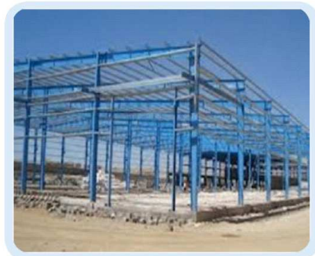
Steel Hangar Building
