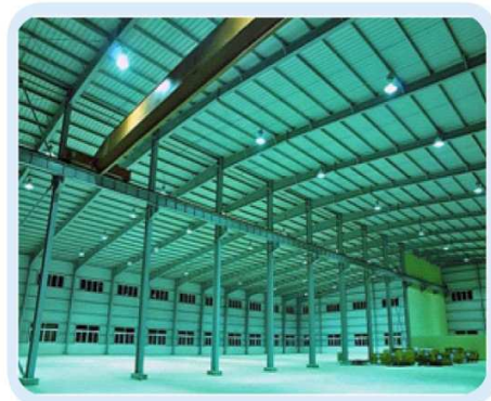
Steel Hangar Building
