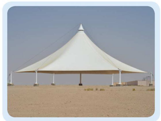
King Khalid City Military Project
